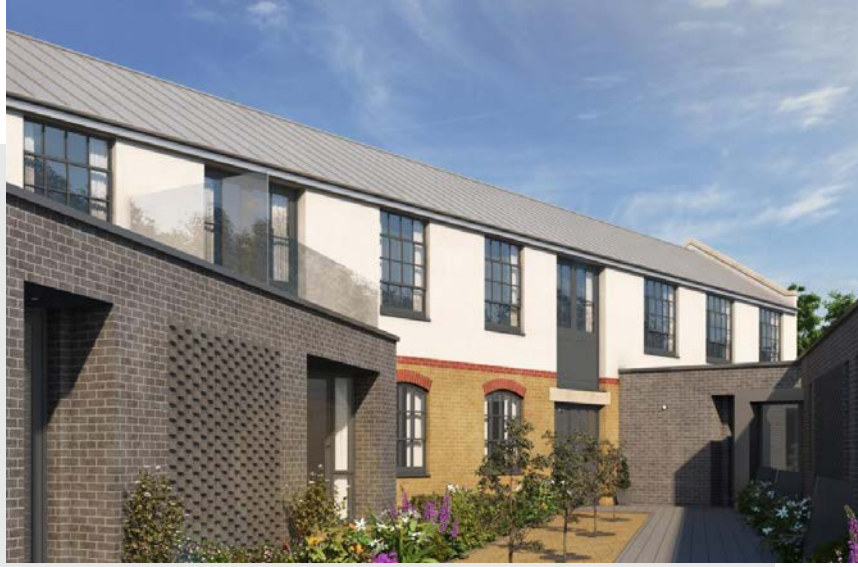
Avignon Road, Brockley
